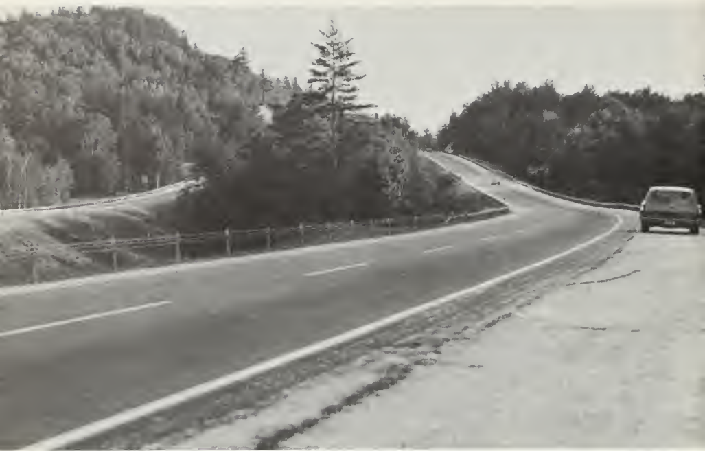
Trees between north and south lanes on this freeway in New York State reduce wind and dust activity, and lower the noise levels, as well as creating a scenic drive.
